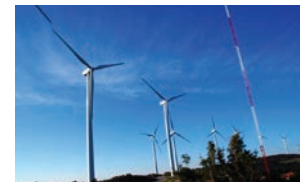
Wind Farm Monitoring (SCADA)
